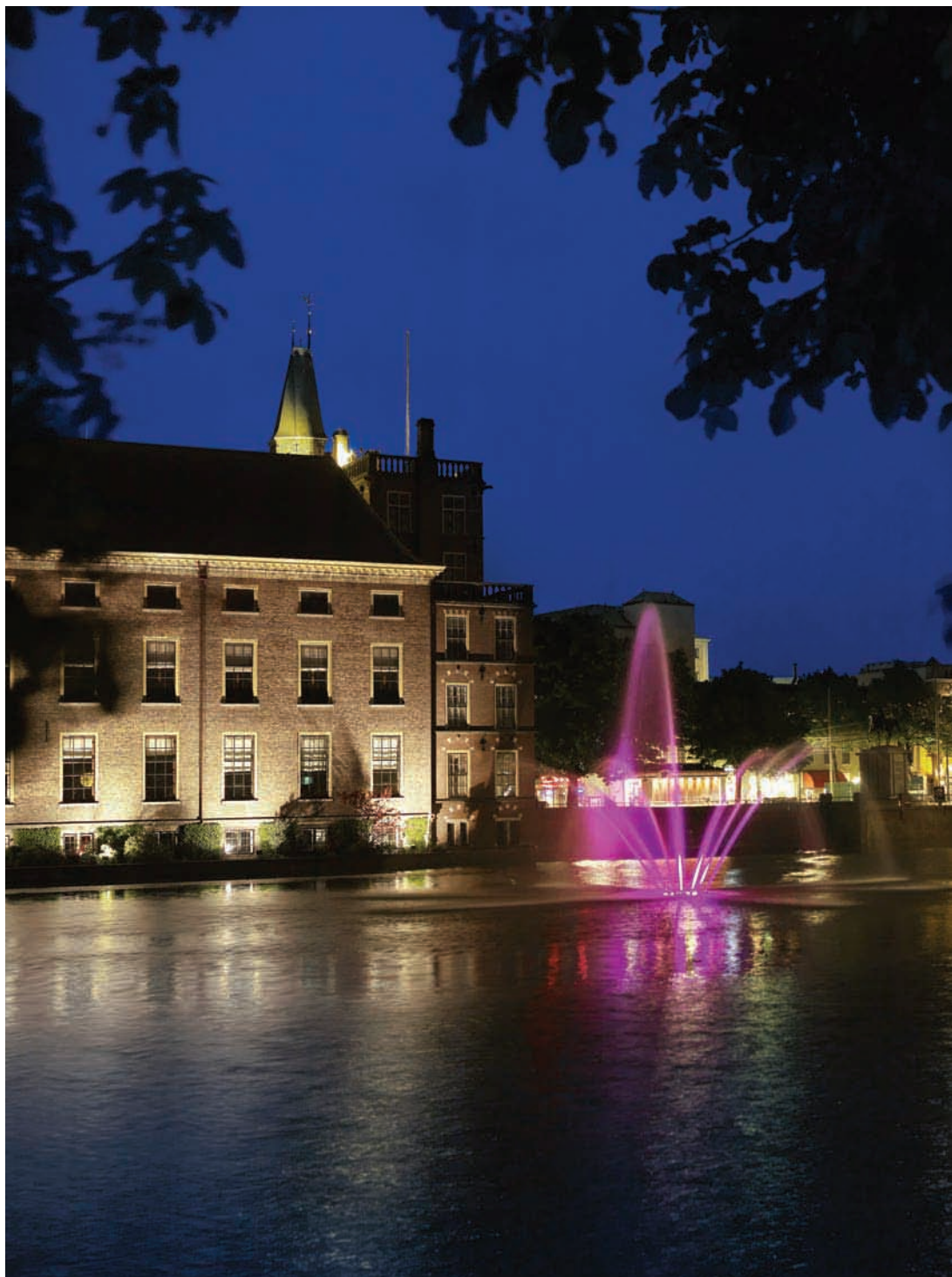
Project: _Helmond Castle, The Netherlands
