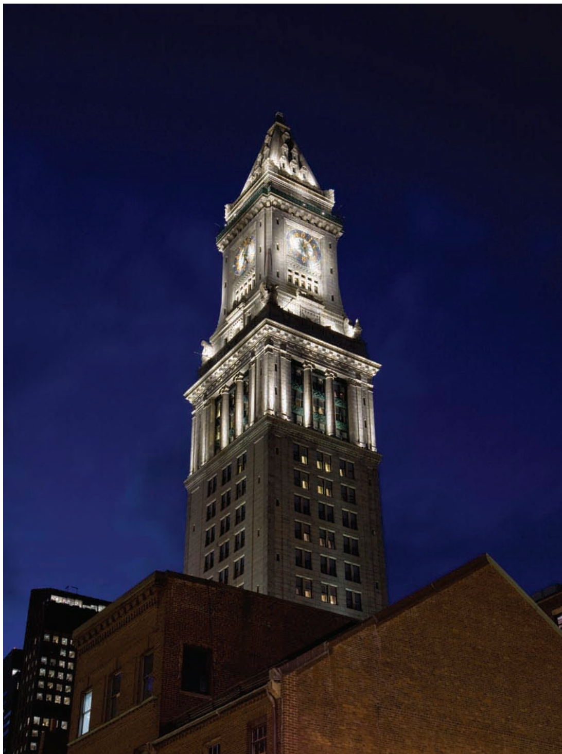
Project: _Custom House Tower, USA Lighting Designer: _Lam Partners Inc.
