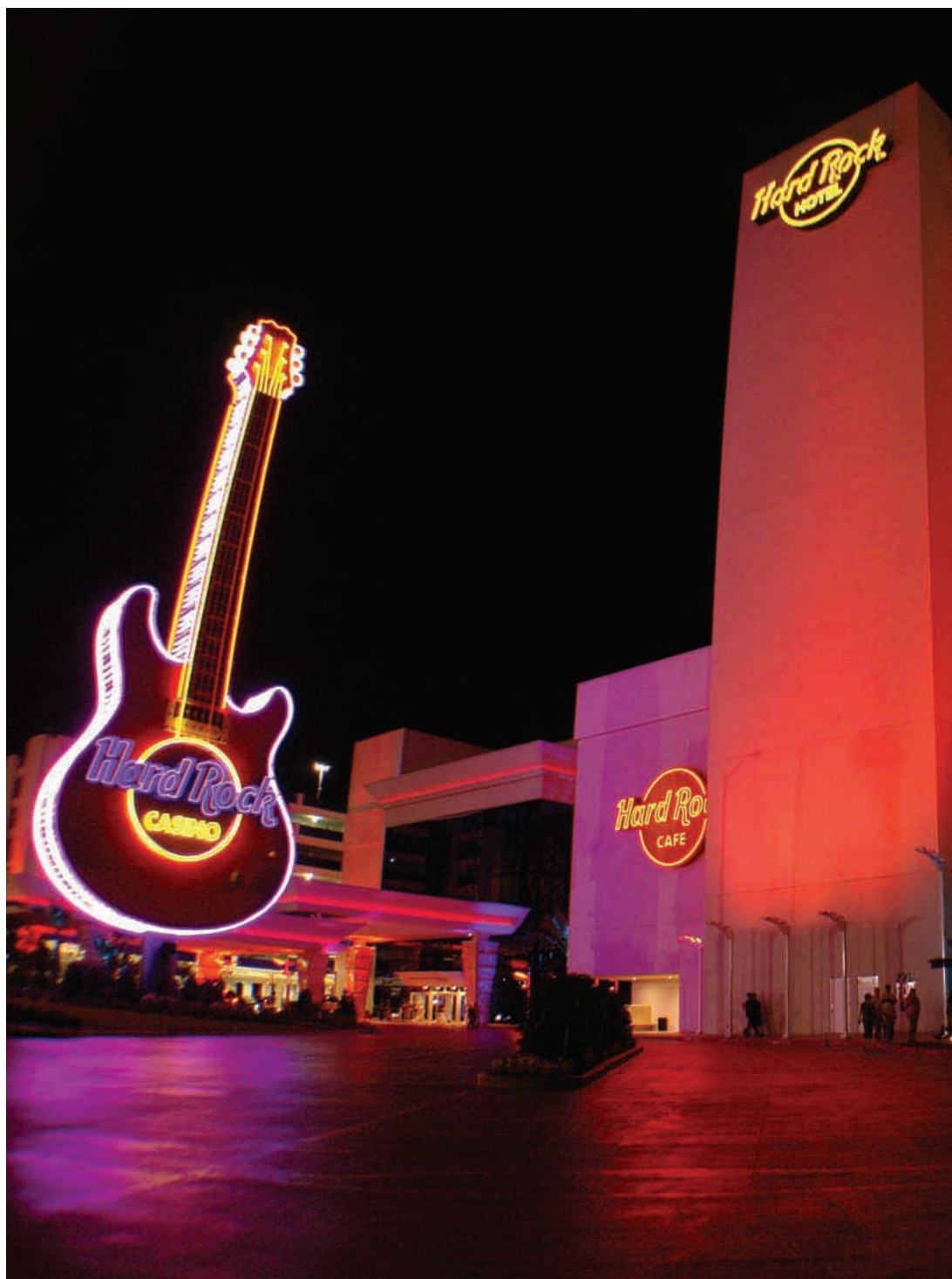
Project: _Hard Rock Cafe Biloxi, USA
